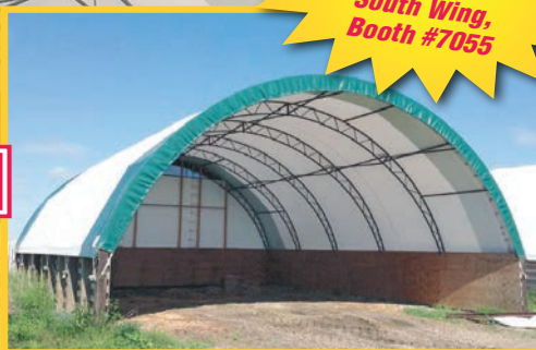
Silver Stream Shelters has been in the hoop manufacturing business for 20 years.
