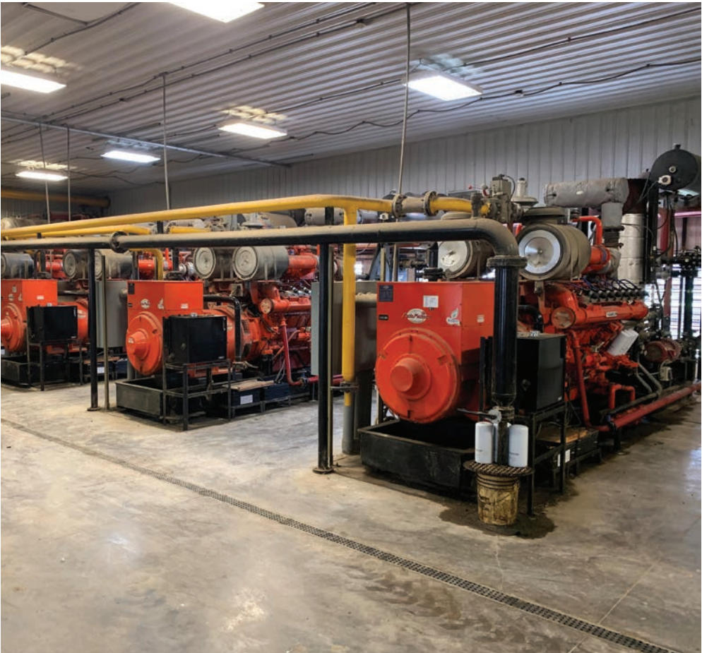
Above: These are the four generators that run on the methane gas.
