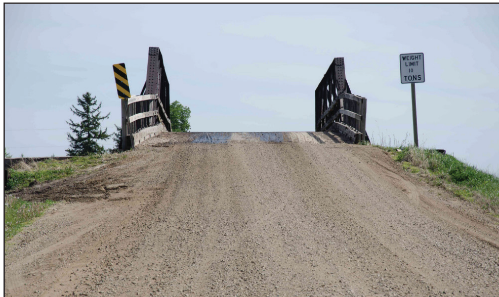
Above: The American Road and Transportation Builders Assoc. recently released its annual "Bridge Conditions Report," highlighting 45,023 bridges in the United States that are rated as 'structurally deficient.' The report said improvement is being made, but much work remains (photo courtesy of Joseph L. Murphy, the Iowa Soybean Assoc.).
