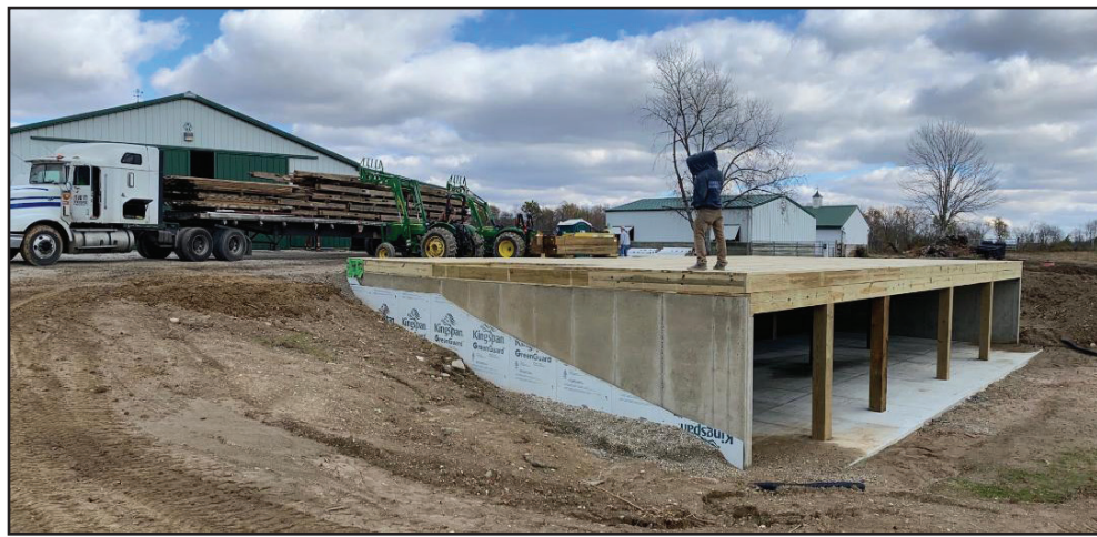
Above: A walk-in basement for delivering calves was dug for the structure of a century old barn moved and pieced back together over the basement.
