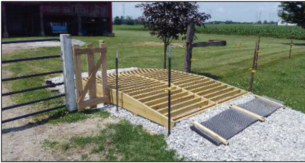
Above: Cows would have to step on an electrified rubber mat if they ever decide to venture across a homemade cattle guard at a farm in Indiana.
