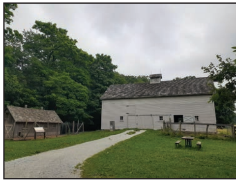
Above: Livestock barn and coop.
