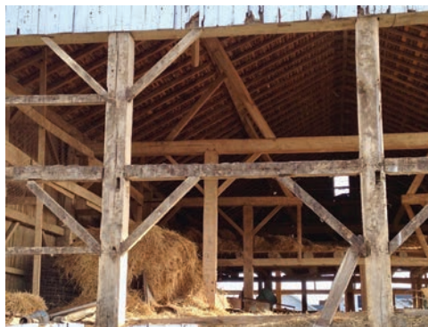
Above: This early- to mid-1800s barn was built with hand hewn logs joined with wooden pegs. It held a corn crib, grain bins, winnowing floor, hay mows, milking stanchions, horse stalls, a hand crank corn sheller and a pioneer-made logging sled. (courtesy of Janet L. Hunter)
