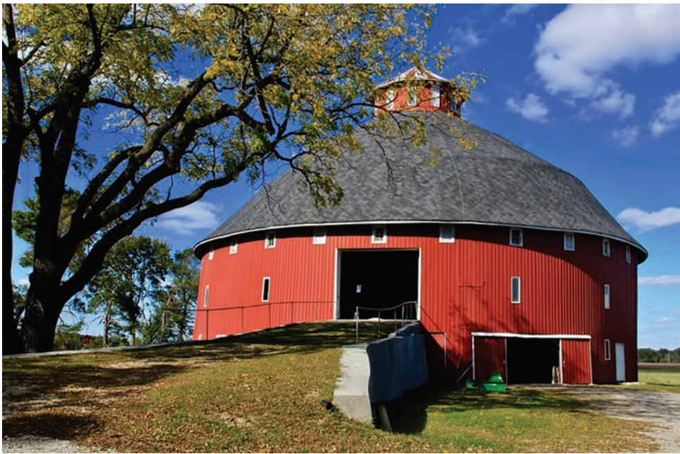
Above: Indiana's largest round barn (shown) was designed by prolific architect and builder Benton Steele in 1903 in Dearborn County, Ind. The diameter of the barn is 102 feet. (photo submitted)
