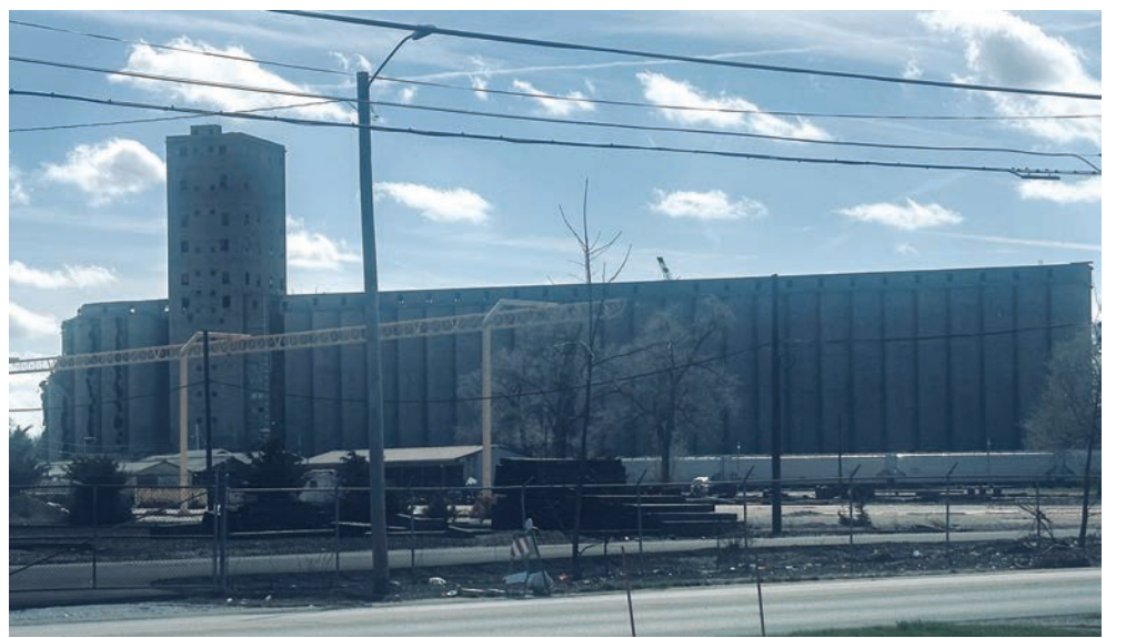
Above: The mill in late March, partially demolished.
