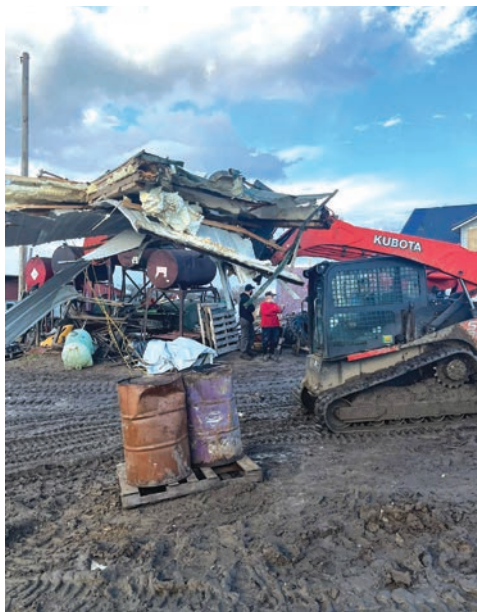
Above: Barns and other outbuildings were destroyed or heavily damaged by a tornado at a family-owned dairy farm since 1963.
