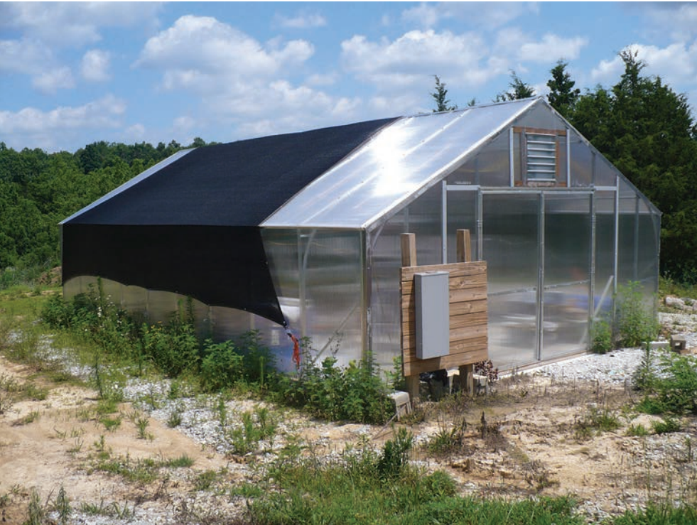
Above: A second greenhouse is being erected on the farm. (photo submitted)
